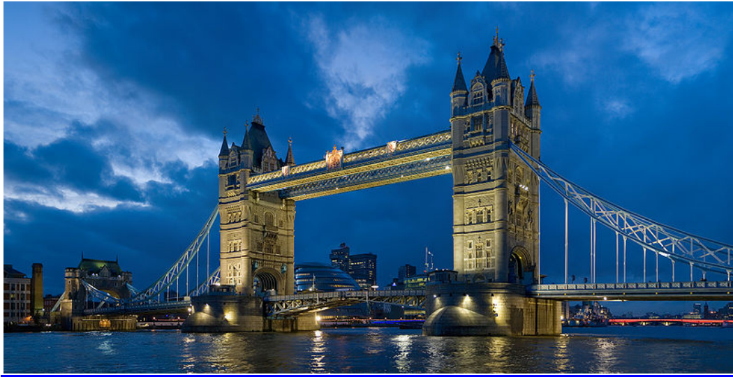
Figure 1 Tower bascule bridge in London, UK [4].
